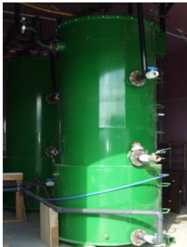
Bio-fuels engineering: anaerobic digester for bio-methane, CO 2 , liquid nutrients, and soil conditioner products from algae
